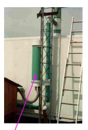
Pump exhaust filter, one of several styles we have used. Our newer pump boxes employ a commercially available filter.
