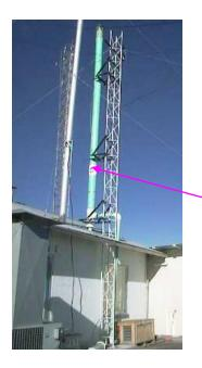
At MLO, the sampling stack is cantilevered away from the tower so that the stack can go through the building roof while the tower attaches to the ground. The access port is 4-5 feet above the roof and can be reached by standing on the roof w/o climbing the tower.
