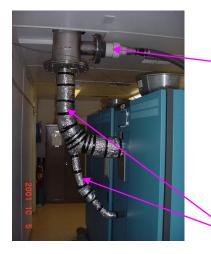
Excess stack flow tube. The pickoff for excess flow can be either inside or outside the building. Air goes to blower in pump shed outside trailer.
