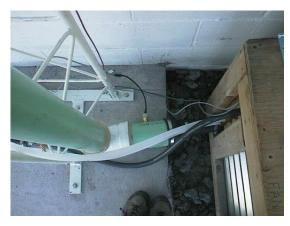
Excess stack flow tube going to pump box outside building. Tower base is bolted to a concrete pad.
