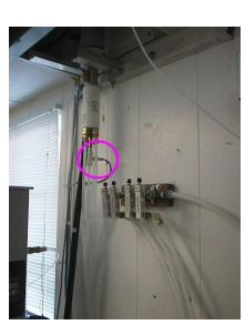
The heater section of the sampling stack goes through the roof of the lab at MLO to the interior. The Vaisala T/RH probe is circled.
