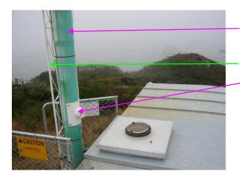
At THD, the sampling stack is attached directly to the triangular met tower. The access port is ~18 inches above the level of the trailer roof. The sampling lines at THD enter the trailer from below, and the excess stack flow line goes to the pump box which is below the trailer.
