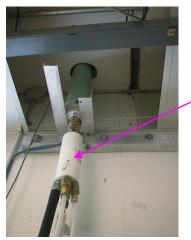
Better view of what comes through the ceiling to the flow splitter. Waterproofing is the key for roof penetration installations.
