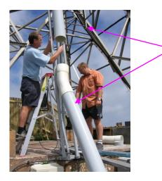
At CPT, the sampling stack is attached to a very tall (60m) tower. The stack has been tilted slightly for an easier entrance into the roof of the laboratory. The access port is easily accessible from the ground (the laboratory was built into the mountain).
