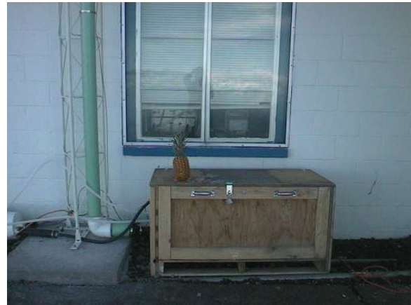
Figure 2-3: Pumpbox at Mauna Loa Observatory. The base of the 10-meter tower and the 10-cm stack bypass line are also seen in the photograph.
