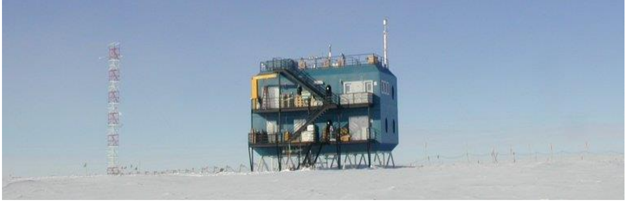
Figure 15. The Atmospheric Research Observatory (ARO) in summer at the South Pole, Antarctica, in which the library is located and two NOAA staff work. Photo by Patrick Cullis, Boulder
