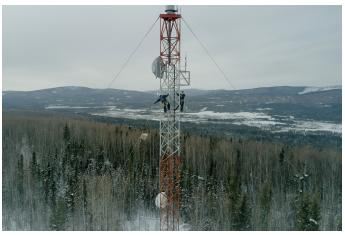
Figure 2. Tower crew installs DCS laser transceivers overlooking Goldstream Valley.
