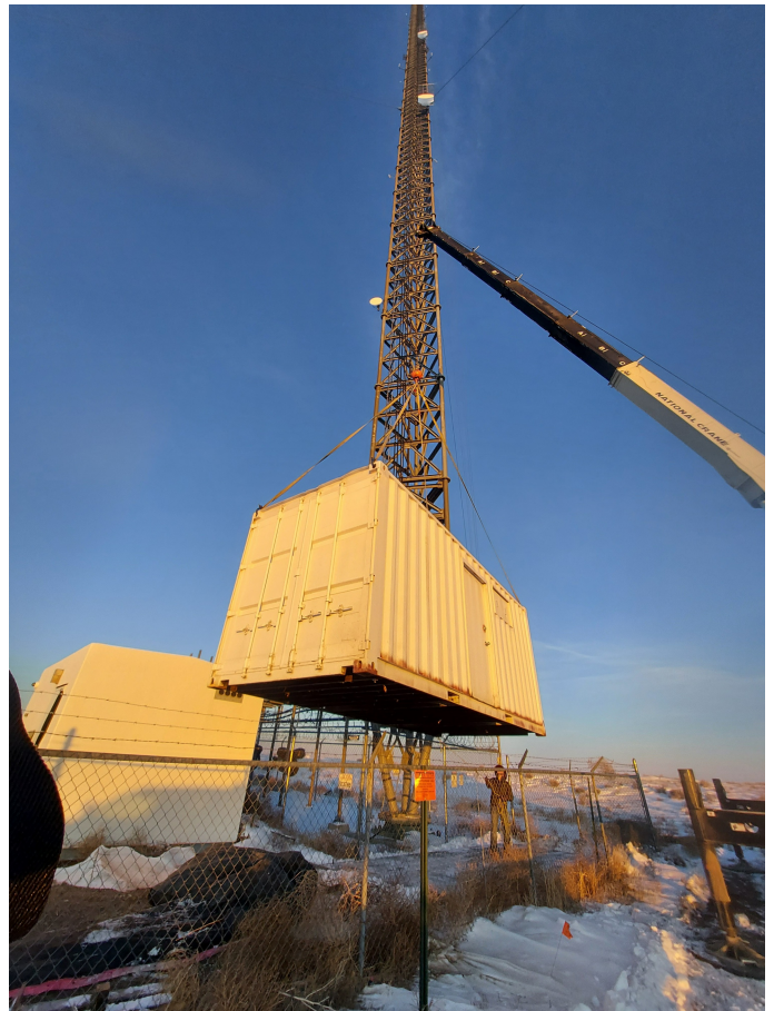
Figure 2. Figure 2. Installing the site container to house instruments and equipment
