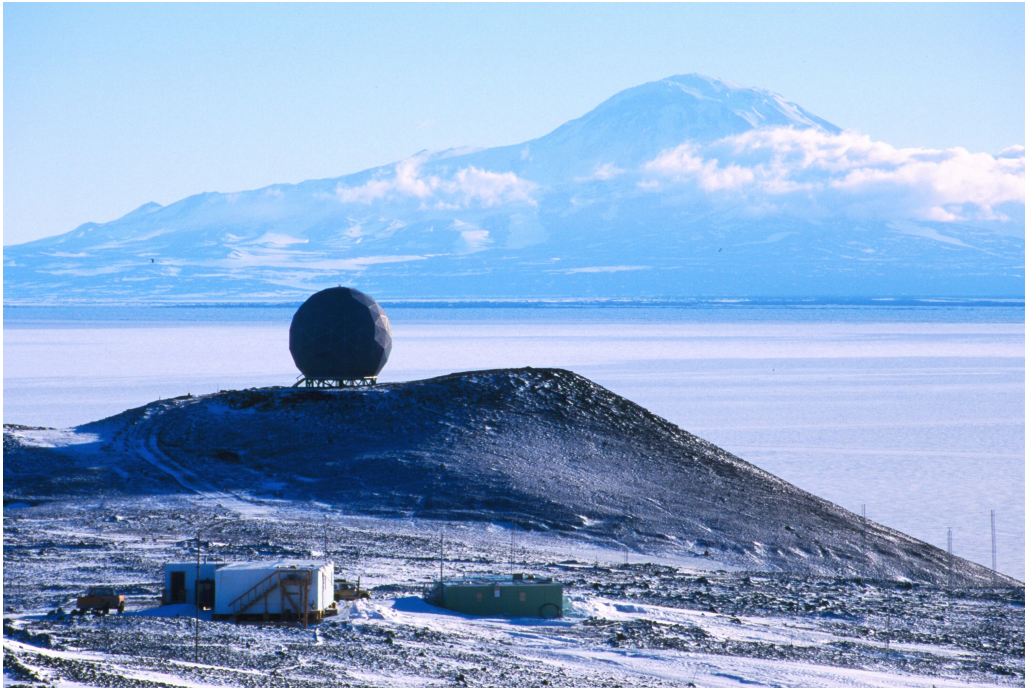
Figure 3.1.1. Arrival Heights in the hills above McMurdo Station. The SUV-100 is installed in the white building in the foreground. The collector is accessible via a stairway that is built on the outside of the facility. The ease of access facilitates maintenance, like cleaning of the collector, and calibrations with the external lamp stand. The green building to the right belongs to the New Zealand Antarctic Program. McMurdo station is located at the foot of the hill, which is marked by the spherical dome serving as a satellite uplink. In the background is Mount Discovery, separated from McMurdo Station by the “McMurdo Ice Shelf.”
