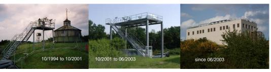
Sites of the BSRN Station. Picture (left): the platform in the first phase (1994 to 2001). Picture (middle): the interim platform during the construction of the new radiation laboratory (2001 to 2003). Picture (right): since June 2003 the BSRN instruments have been installed on the roof of the radiation laboratory, at the site of the first platform.
