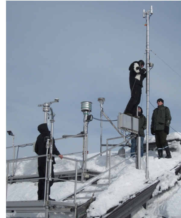
Installation of separate inlet line at Pallas
