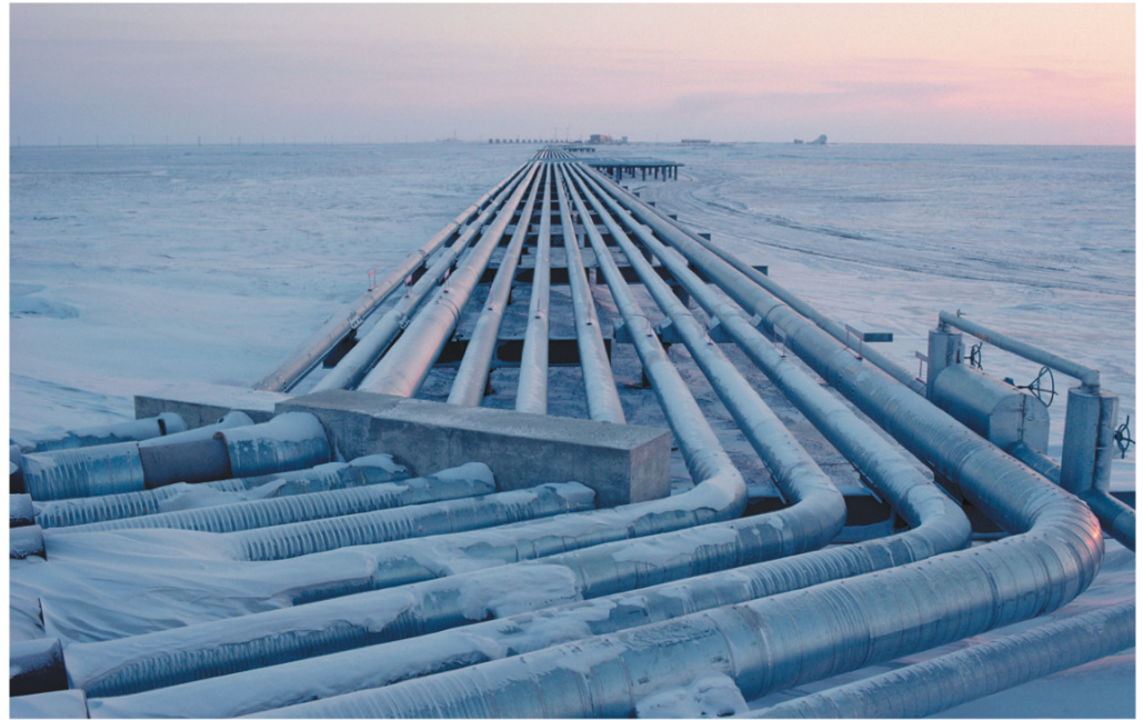
Pipes transport oil from rigs on Endicott Island in Alaska.
