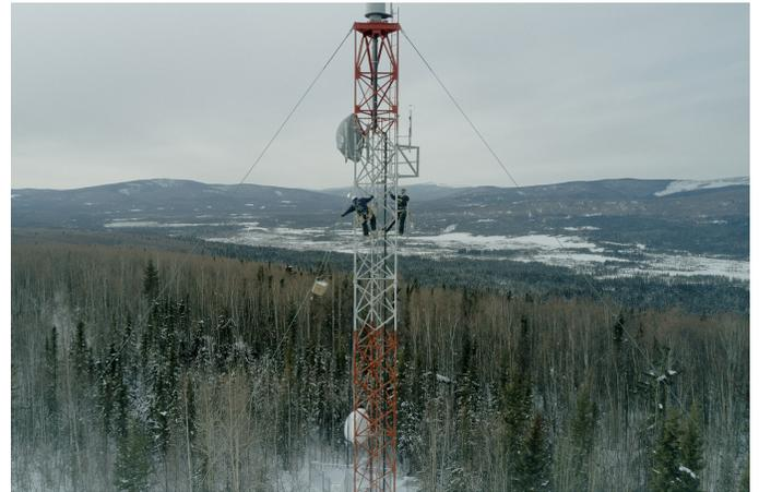
**Figure 2.** Tower crew installs DCS laser transceivers overlooking Goldstream Valley.
