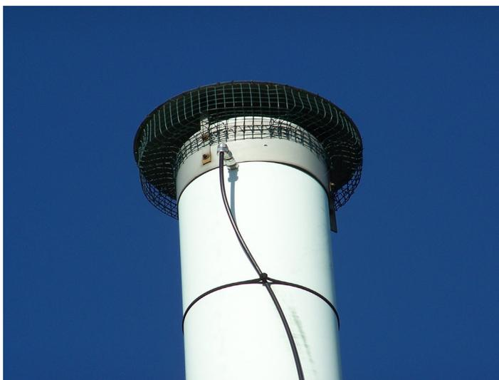
Fig. 3-3a: (a) Old-design sampling stack rain cap.
