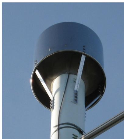
Fig. 3-3b: (b) New-design sampling stack rain cap.
