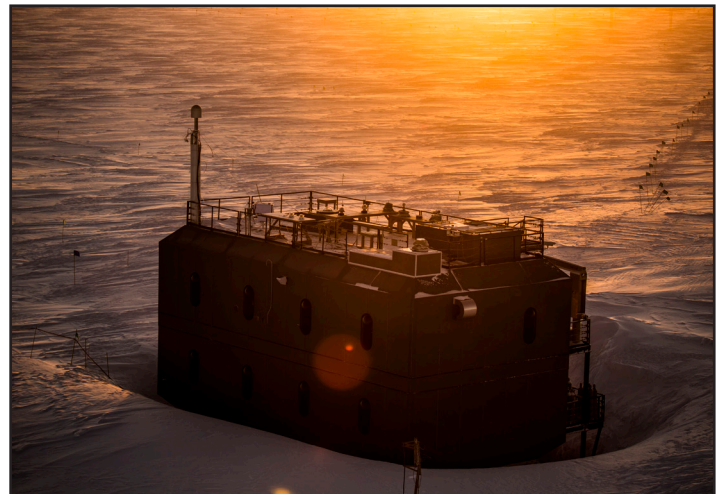
Figure 2:16: South Pole Atmospheric Research Observatory in a hollow of drifted snow in late winter viewed from the meteorological and sampling tower.
