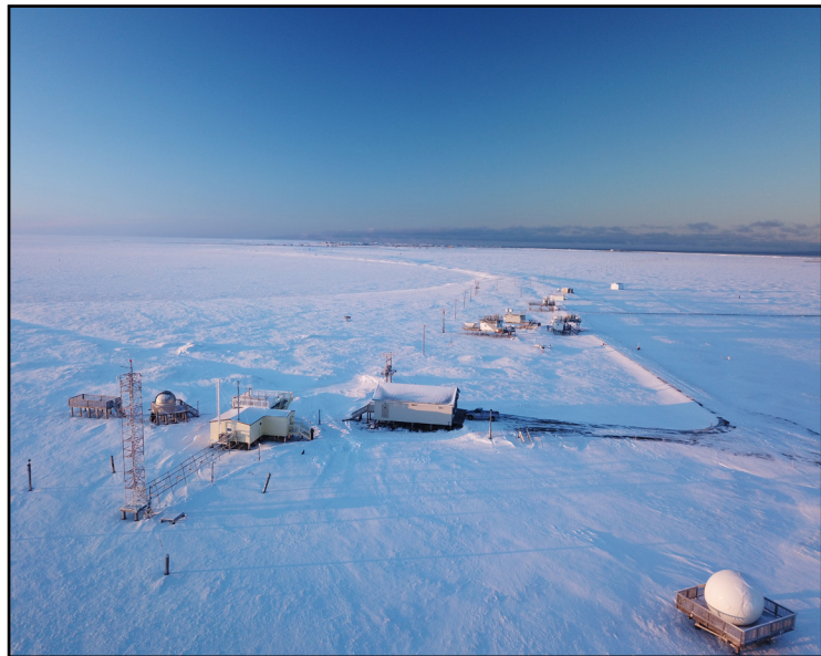
Figure 2.1: Barrow Atmospheric Baseline Observatory compound with the Department of Energy facility in upper right center and NESDIS Polar Orbiting Satellite downlink antenna in the lower right in winter.
