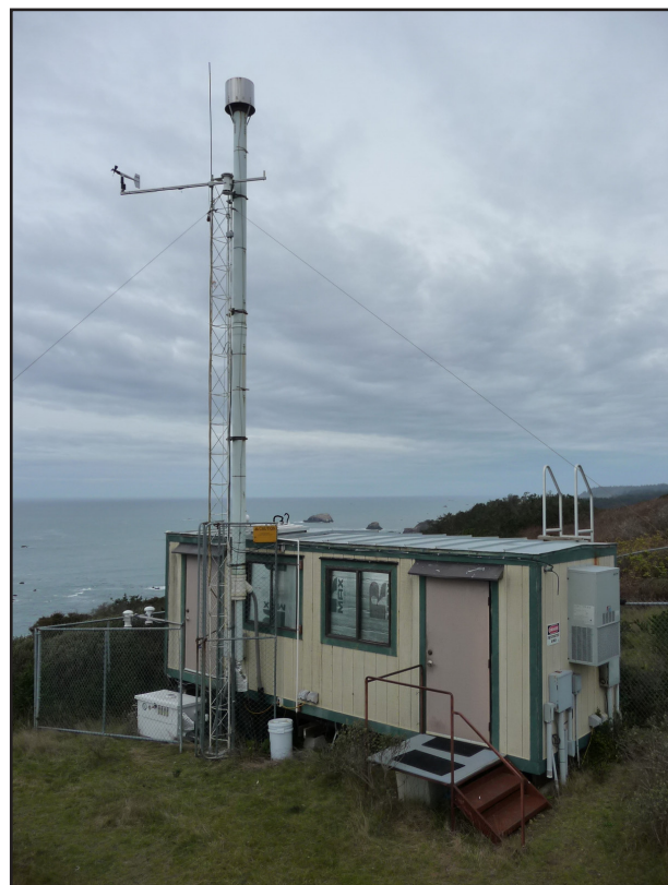
Figure 2.5: Trinidad Head Observatory building located on the west side of the Head facing the Pacific Ocean.
