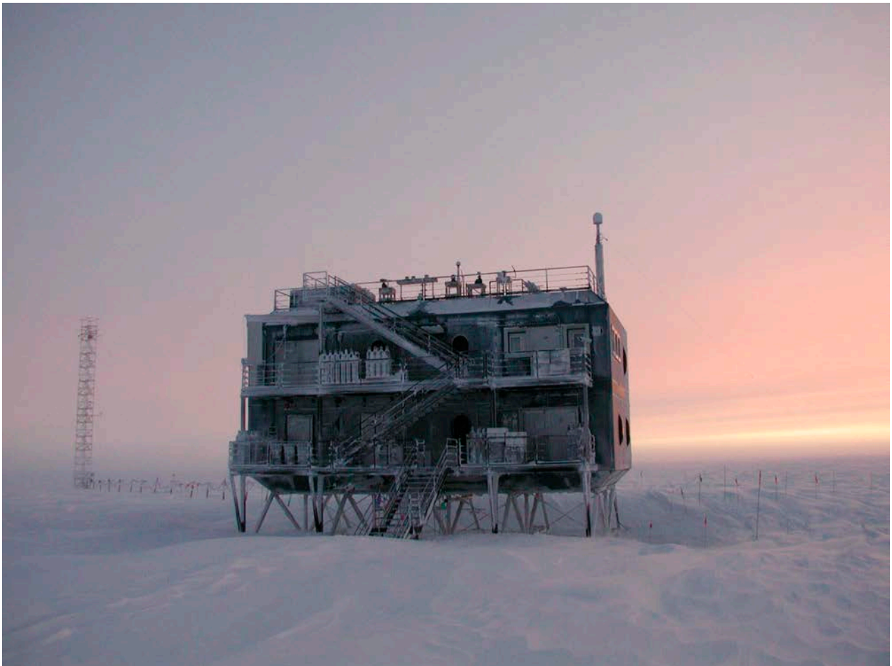
South Pole Observatory
