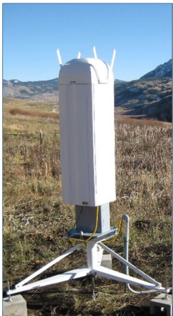
Ceilometers installed at SURFRAD & mobile deployments
